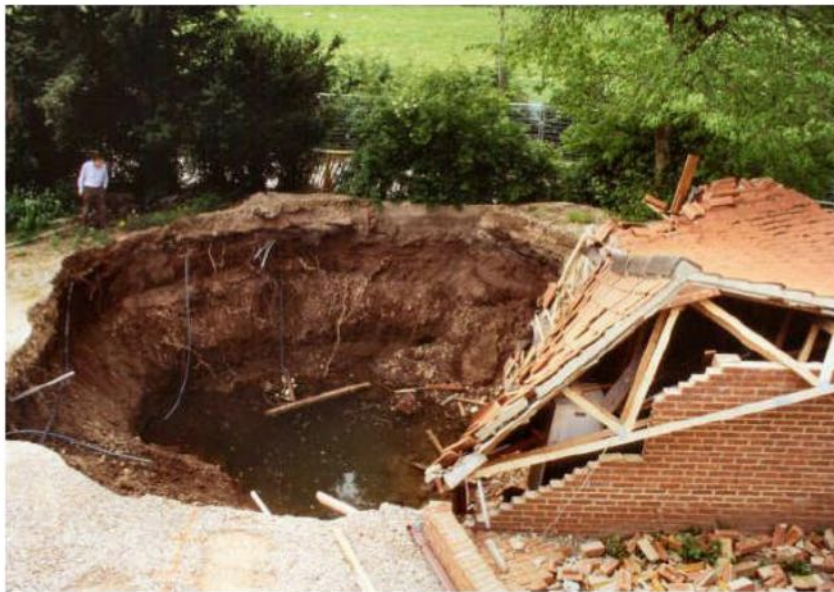
Figure 3-1 Ure Bank Terrace, Ripon sinkhole collapse, April 1997, reproduced from Cooper 2007
