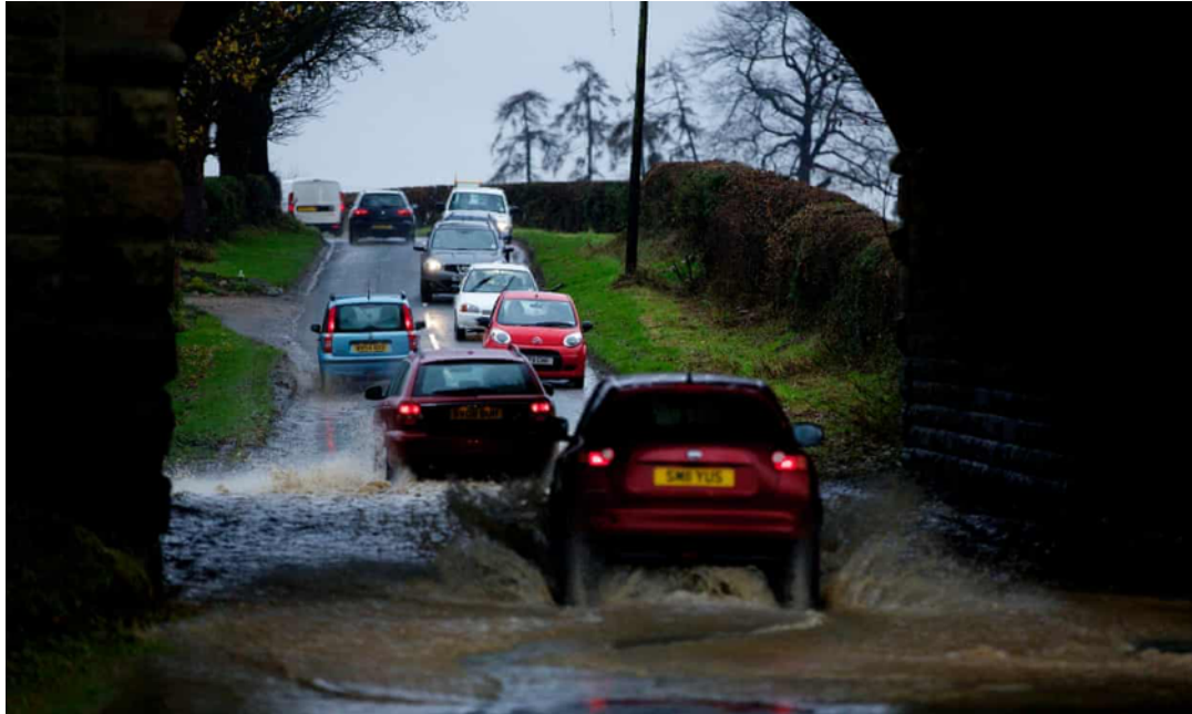
C377 route towards Ripon flooded beneath the bridge (November 2012).
