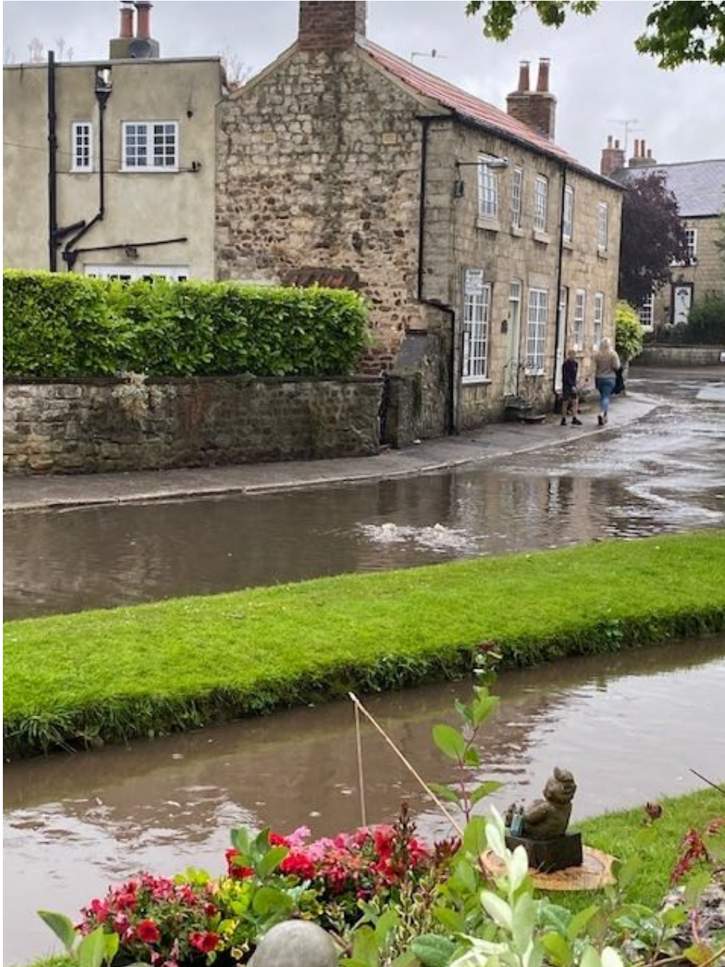
Figure 4 – Further view of the same village-centre incident, showing the escape while the Beck remains within its channel.
